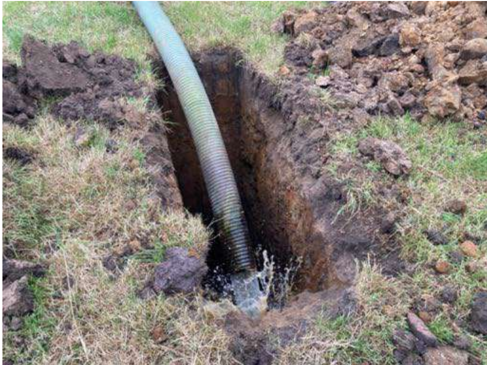
Photograph 13 Description: Discharge of water into trial pit TP01 Date: 20/07/2022
